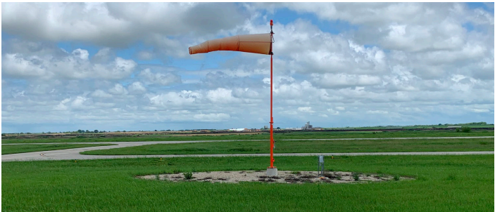
Primary Wind Cone and Segmented Circle
