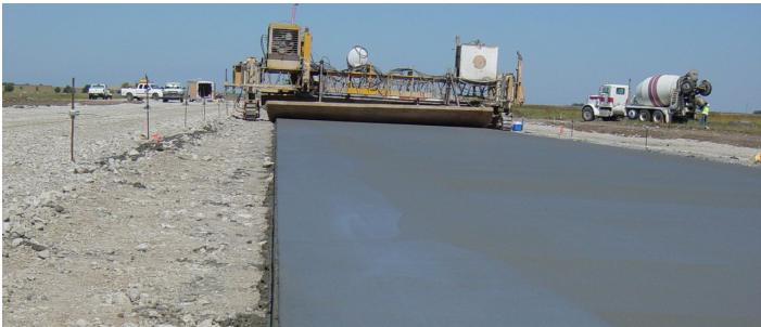
Runway 17-35 Paving Operations
