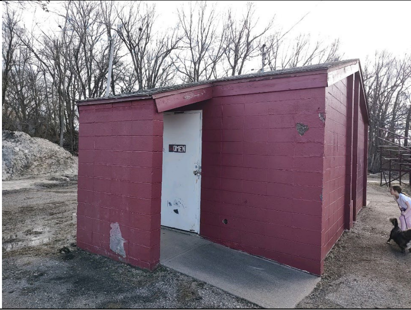
Women's side Wall repairs where fountain was on north side.
